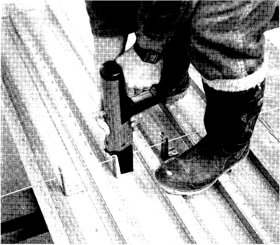
Fig. 21.11 Shot-fired shear-connector
