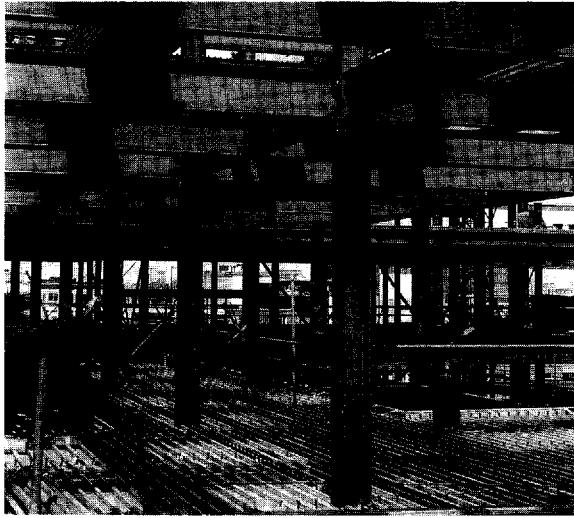
Fig. 21.2 Composite building under construction showing decking and shear-connectors
