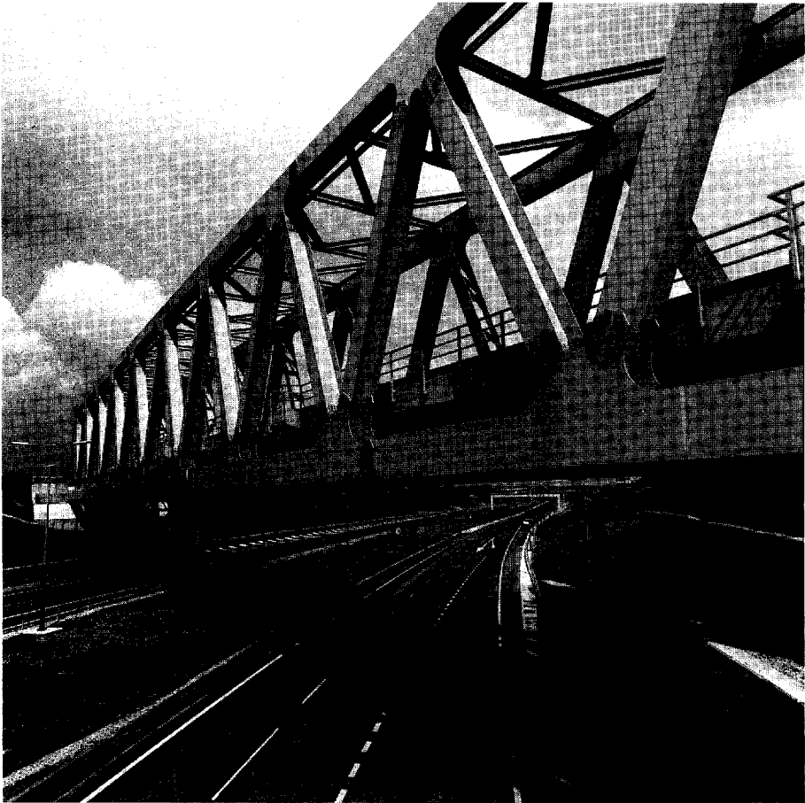
Fig. 19.2 Brinnington Railway Bridge
